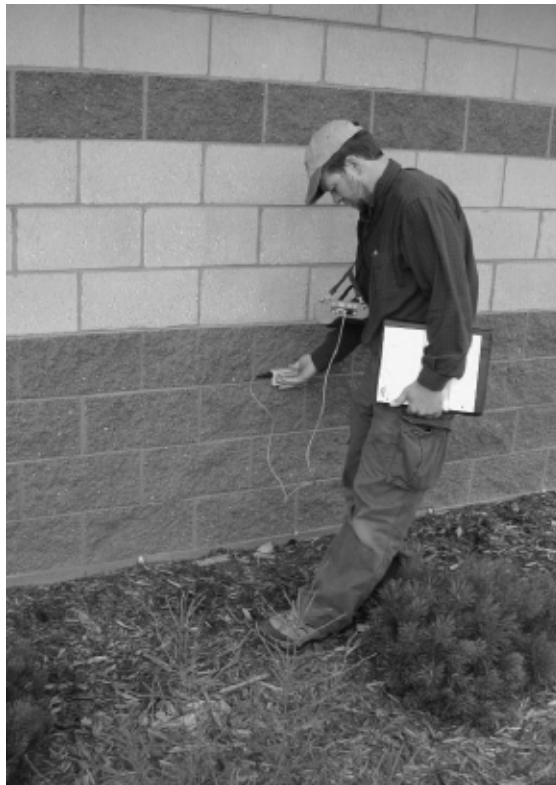
Fig. 14. Finding reinforcement location using an eddy current induction metal detector.
