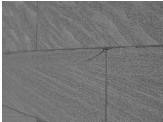
Fig. 4. Incipient spall in limestone.
