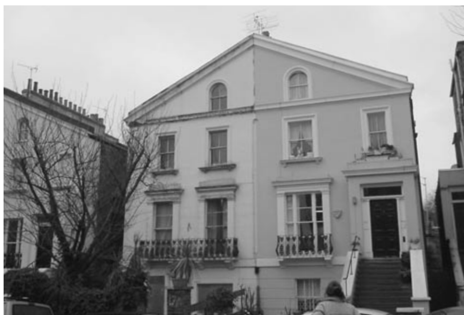
Fig. 1. The Low Energy Victorian House (LEVH), in Camden, north London, is the left half of two semi-detached properties. All photographs by Bob Lowe and Ian Ridley, Bartlett School of Graduate Studies, University College London.
