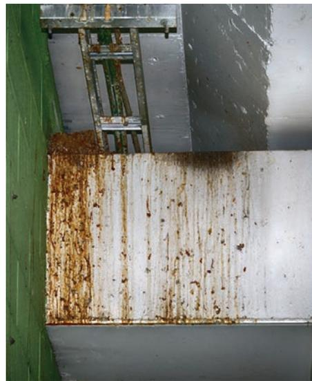
Fig. 5. Grain silo, Holbrook, Australia, showing accumulation of pigeon excreta at a nighttime roost.
