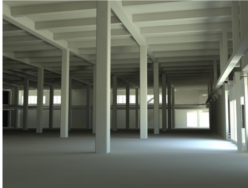
Interior view of the structural members within the May Co. Building BIM
